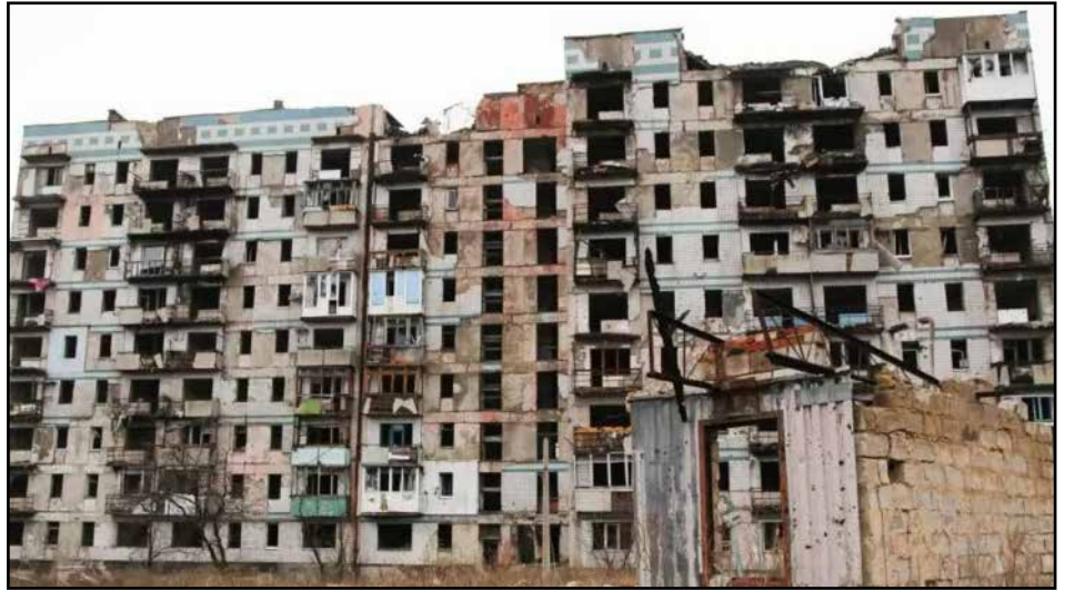
Donbass Buildings destroyed
